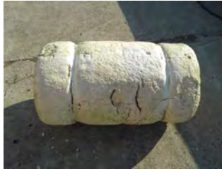
Inside Polystyrene Foam
