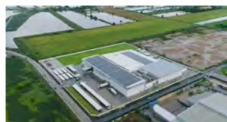
Solar Power Generation Facilities (Thai Delmar Co., Ltd.)
